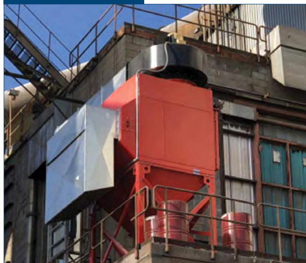
Self-maintaining air cleaner installed on exterior of steel mill.
