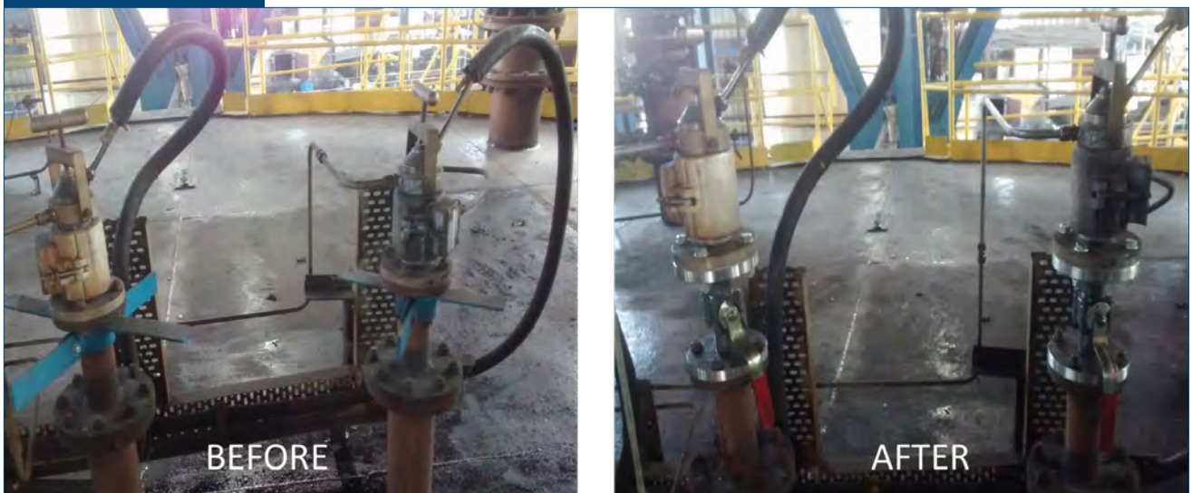
Installation of new designed probe with isolation valve in coal injection plant.
