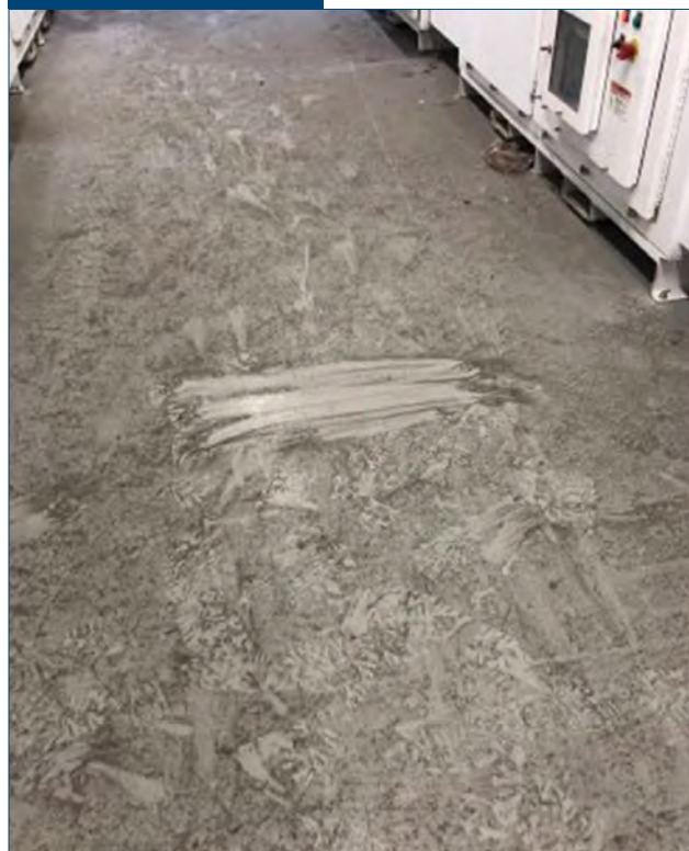
Dust accumulation in a motor control center.
