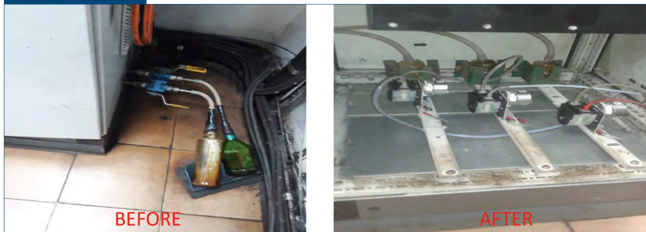
Manual collection of condensate in bottles vs. automatic draining of condensate.
