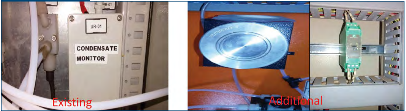
Redundancy built up of condensate monitor in top gas analyzer.
